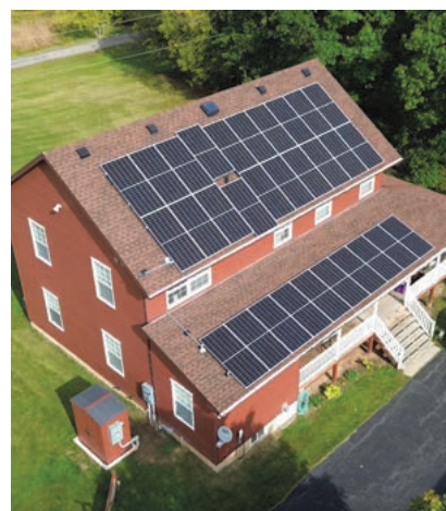
SIX NATIONS SOLAR POWERED OFFICE © COURTESY OF PLENTY CANADA
